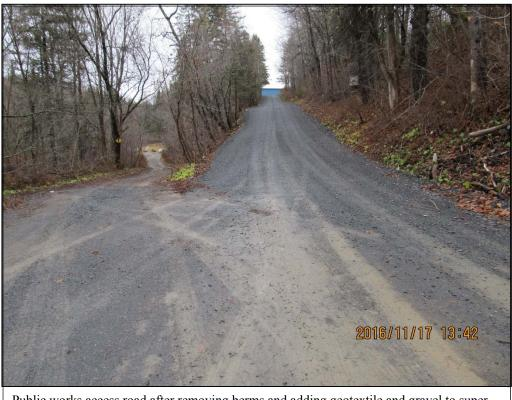
Public works access road after removing berms and adding geotextile and gravel to superelevate the road. Reshaped ATV trail and used large rocks to restrict ATV access.
