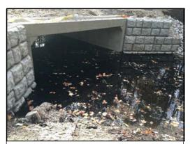
Kala Lane - The Town replaced two undersized culverts with a concrete box culvert with natural bottom.
